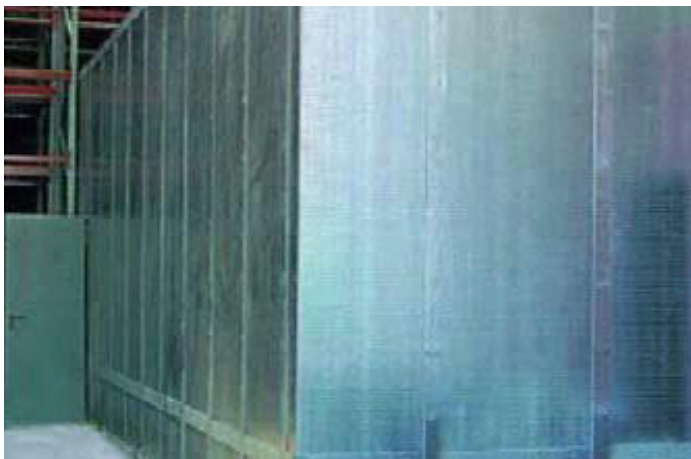
An Acoustic Enclosure
